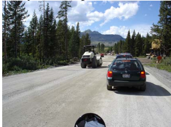
9 miles of muddy, gravel road construction
